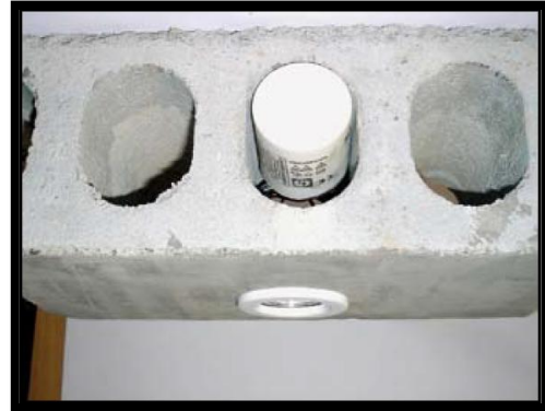
Figure 12 - Example of down light in hollow core plank
